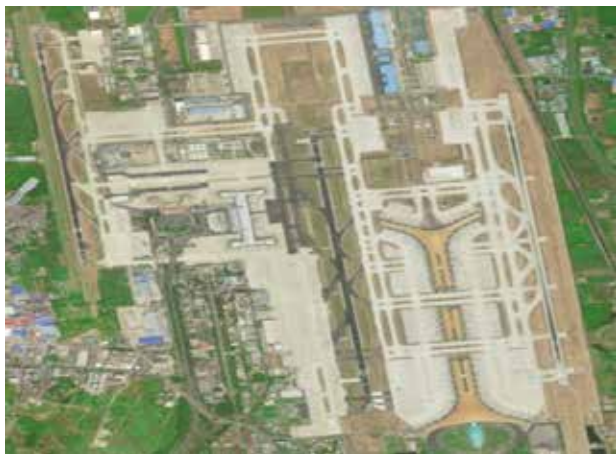
Figure 2- Satellite Image of Beijing T3 Terminal Building
